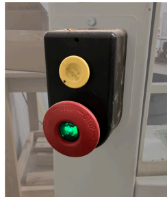
Figure 6: Resaw band saw power switch.
